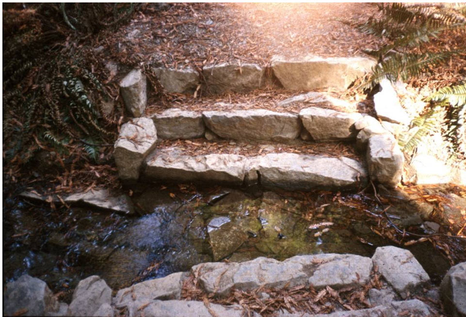
Photo 14.8 - Step Through Culvert
