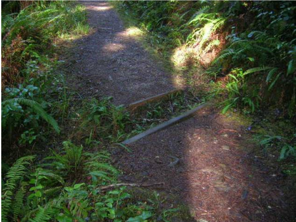
Photo 14.10 - Open Wooden Culvert
