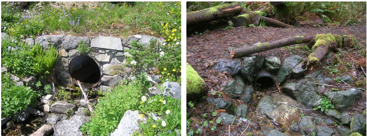
Photo 14.12 - Metal Culvert (left), Plastic Culvert (right)
