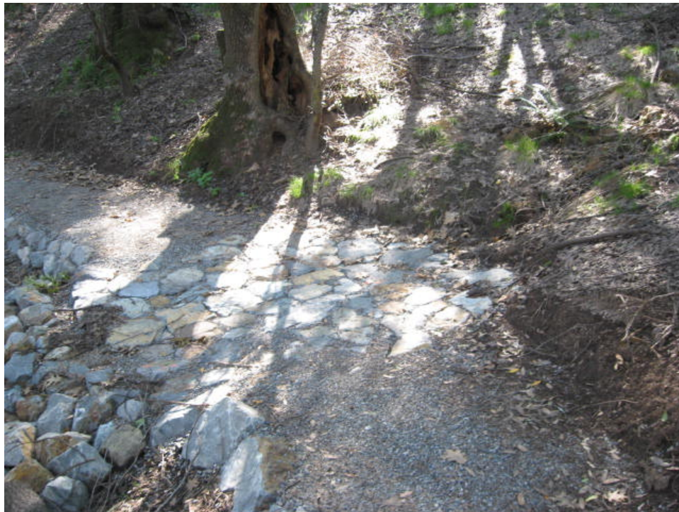
Photo 14.4 - Armored Drain Swale
