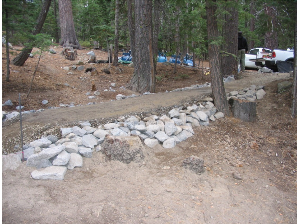
Photo 14.16 - Drain Lens
