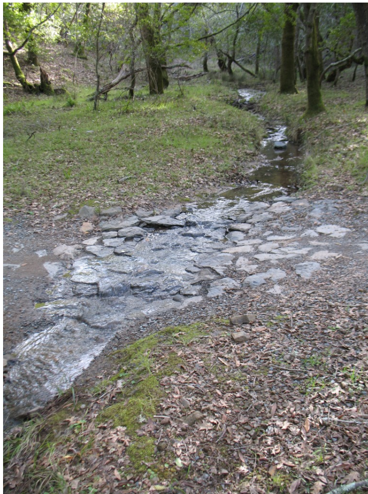
Photo 14.5 - Armored Stream Crossing
