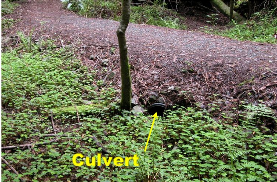
Photo 14.17 - Drain Lens with Culvert
