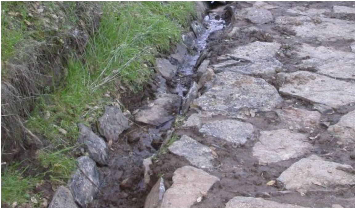
Photo 14.6 - Drainage Ditch
