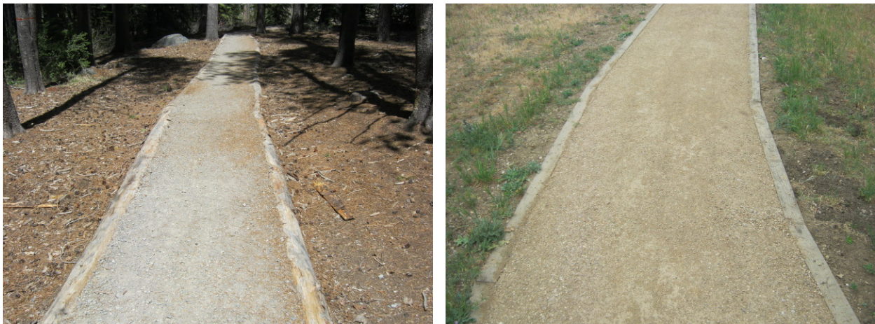
Photo 14.18 - Log Turnpike (left), Lumber Turnpike (right)
