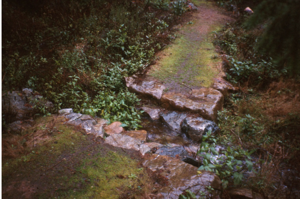
Photo 14.7 - Open Rock Culvert
