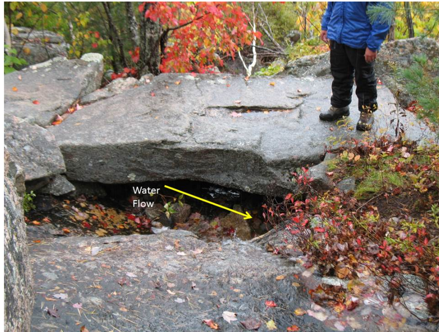
Photo 14.9 - Closed Rock Culvert
