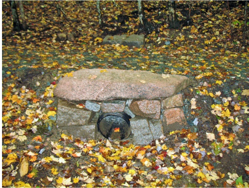
Photo 14.13 - Culvert Headwall
