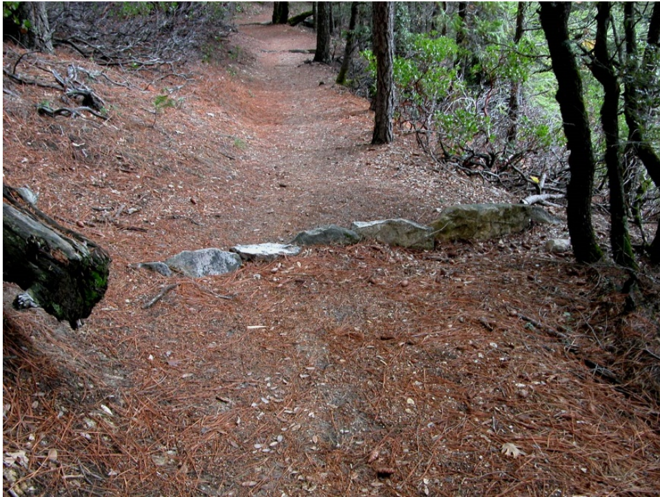
Photo 14.20 - Rock Water Bar
