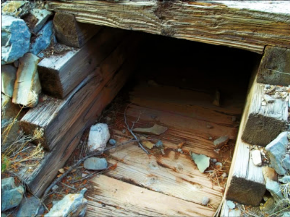
Photo 14.11 - Wooden Culvert
